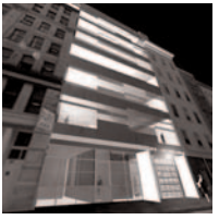
31-33 Vestry Street Architectonics, 2006
