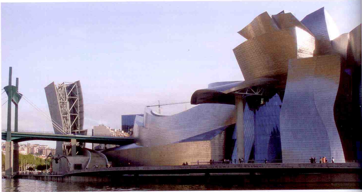
The Guggenheim Museum Bilbao Frank Gehry, 1996 Photo: The Guggenheim Museum
